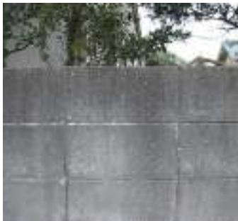
Before/洗浄後施工
